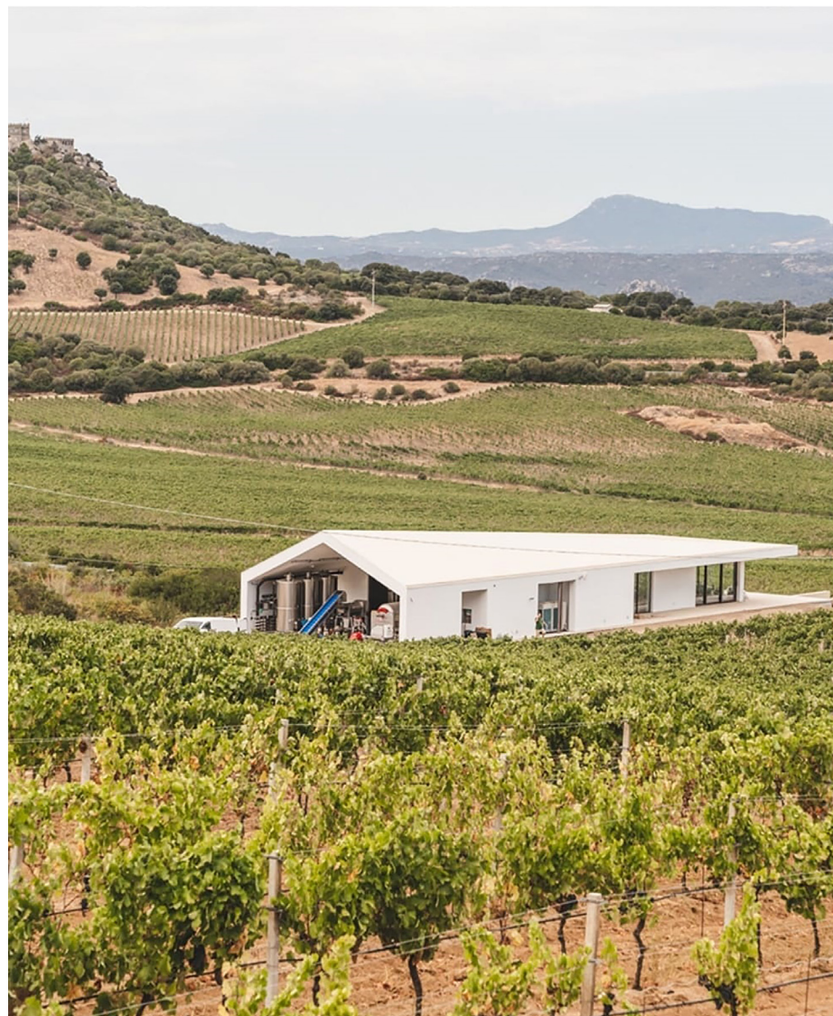
Cantina vinicola, Loiri Porto San Paolo, 2019-2021
